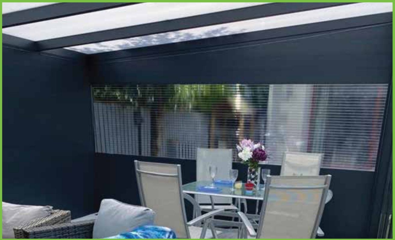
Here is an example of a veranda sidewall fitted with 1/2 and 1/2 Ultra Clear polycarbonate panel and Aluminum sidewall.
